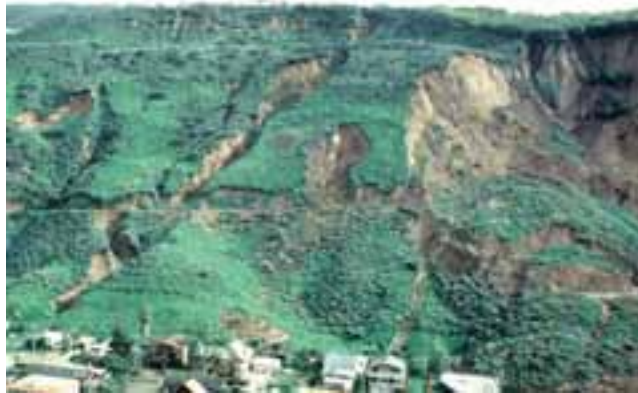
Figure 6.6: 1994 landslide (USGS photo).
