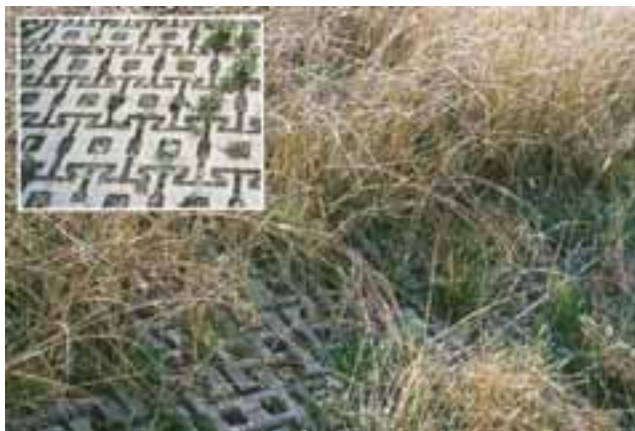
Figure 5.17: Soil surfaces may be covered with products that provide strength for slope stability and still allow water to infiltrate and plants to grow.
