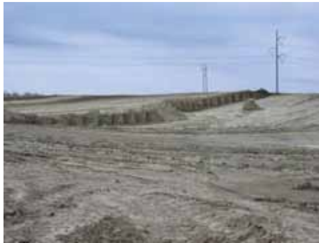
Figure 3.13: A cut on a construction site. This site is subject to wind erosion.
