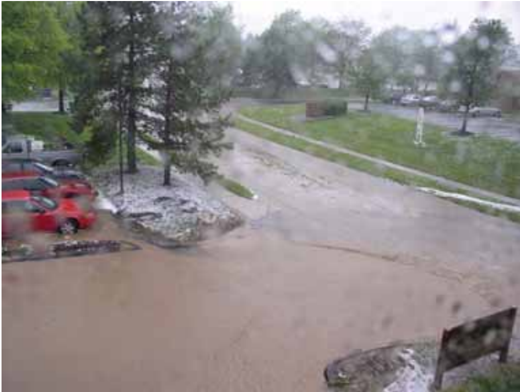
Figure 3.12: A flooded parking lot and street.
